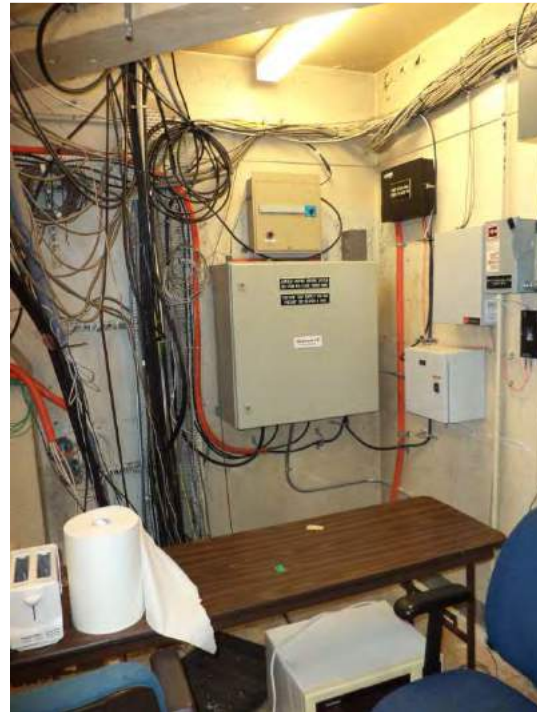
Break room/mechanical room
