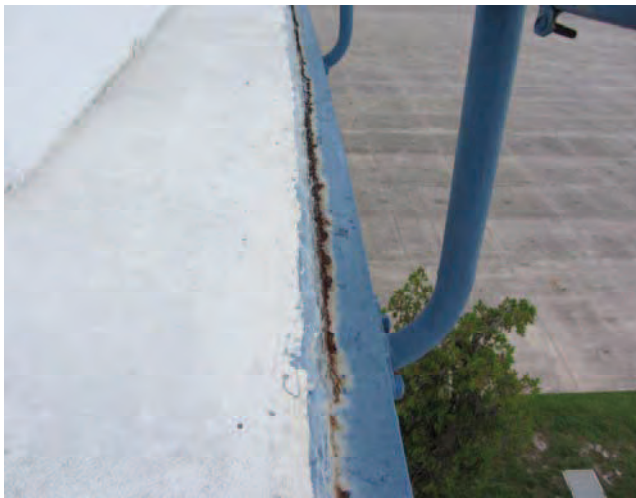
PICTURE 15 – Rusting at Main Level Railing of Control Tower
