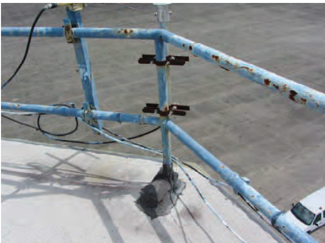
PICTURE 18 – Rusted Railing at High Roof Over the Cab
