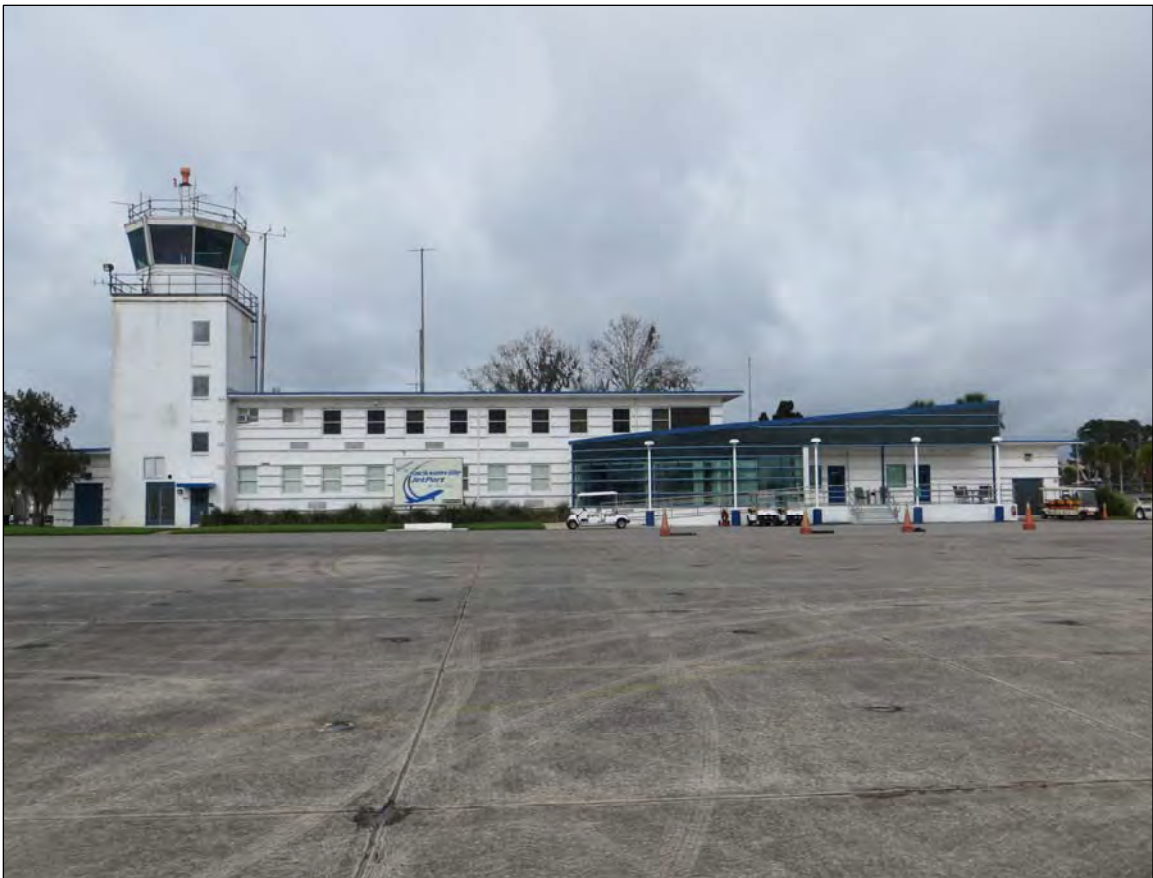
Figure 6. Resource 8DU21750, Cecil Airport Traffic Control Tower, facing northeast (top left), facing northwest (top right), facing west (bottom).
