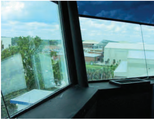
PICTURE 13 – Typical Support for Control Tower Roof/Glazing System
