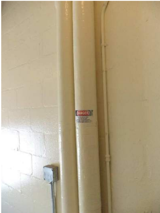
ACM label on pipe insulation in stairwell
