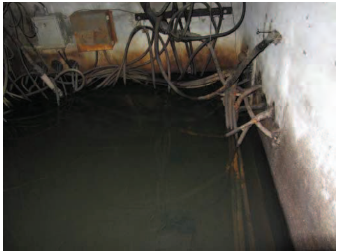
PICTURE 4 – Pit View With Standing Water
