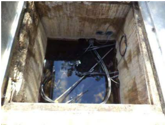
Vault with water intrusion
