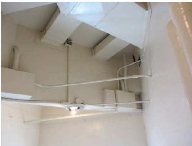
PICTURE 11 – Ductwork Through Walls
