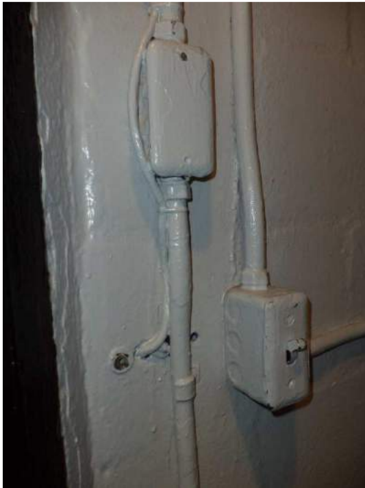
Typical electrical fixture
