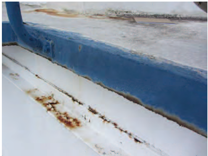
PICTURE 16 – Rusting at Main Level Railing and Support Angle of Control Tower
