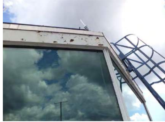
Cab roof access
