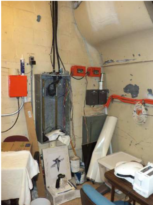
Break room/mechanical room
