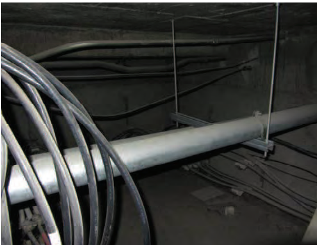
PICTURE 5 – Power / Cable Vault
