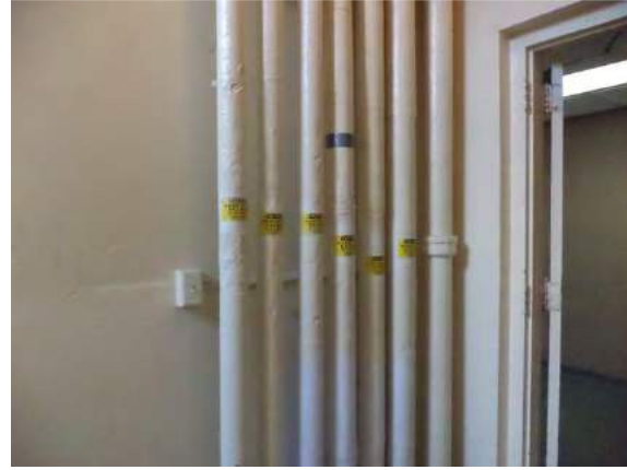
ACM labels on pipe insulation in stairwell
