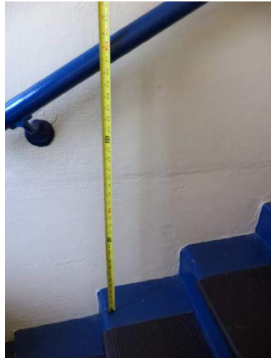
Handrail in stairwell
