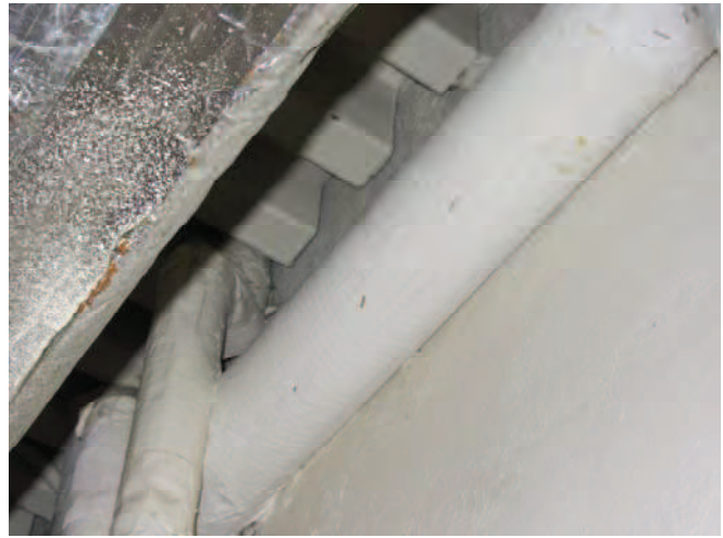
PICTURE 8 –Floor Deck Does Not Extend to Bearing Wall
