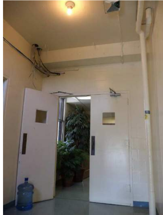
Stairwell door at 2 nd level
