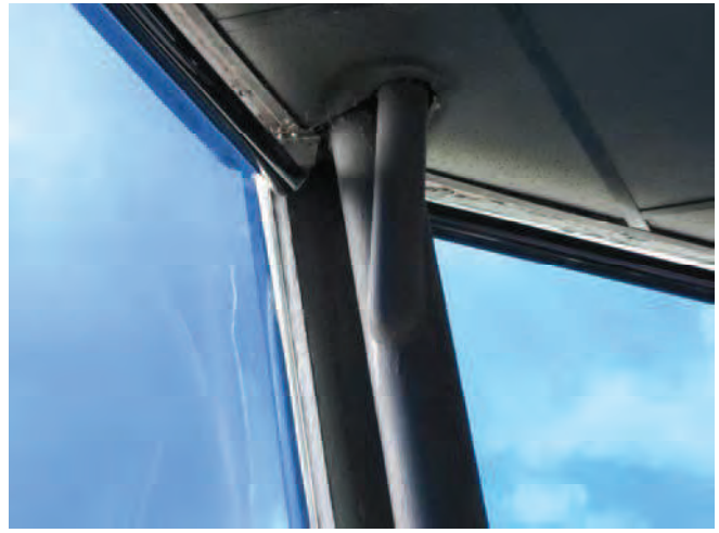
PICTURE 14 – Typical Bracing at Top of Control Tower Support
