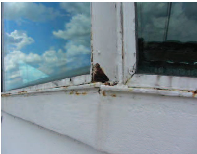
PICTURE 17 – Rusting at Base of Control Tower Window
