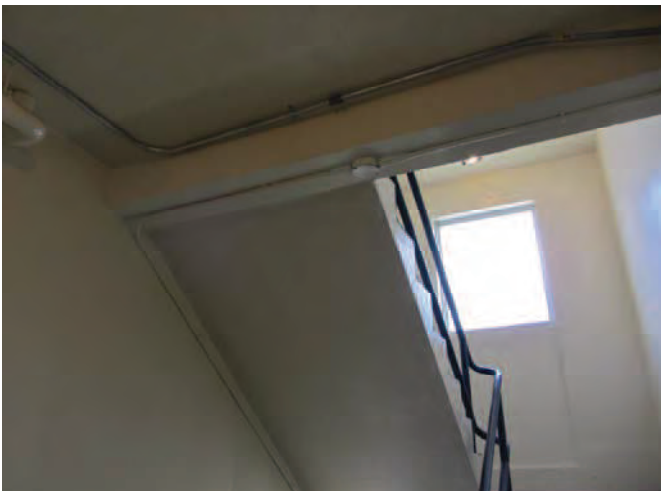
PICTURE 6 – Framing for Stair System
