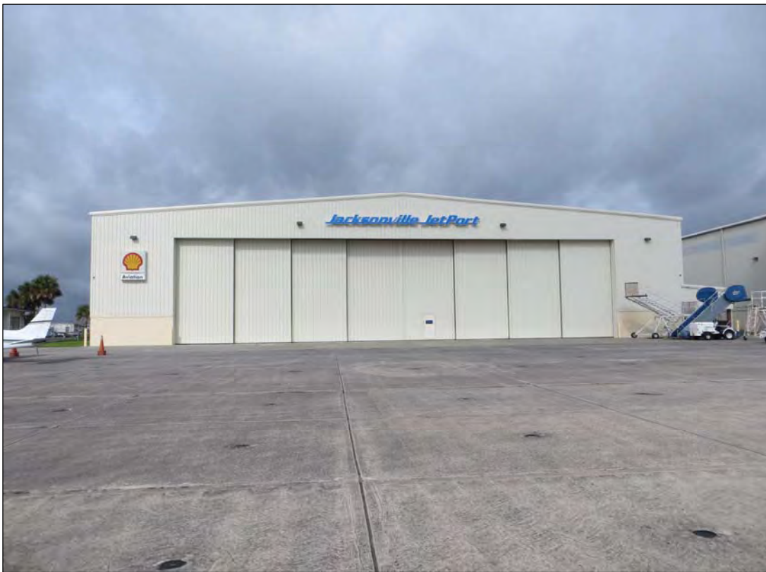
Figure 7. Modern hangar, built in 2012 just north of Resource 8DU21750, overview with tower in background (top), east elevation (bottom).
