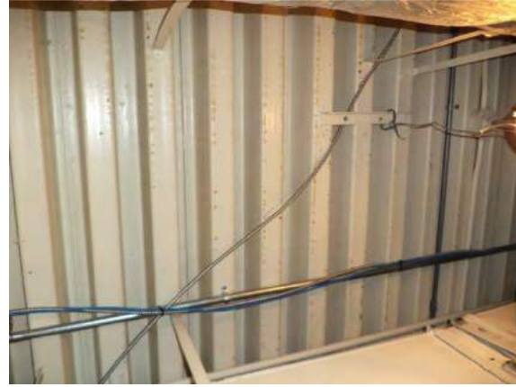
Structural deck at wall with water intrusion
