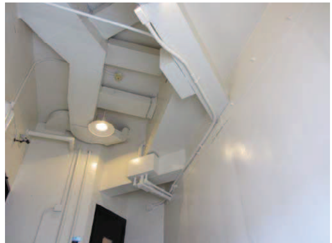
PICTURE 10 – Control Tower Cab Support Framing
