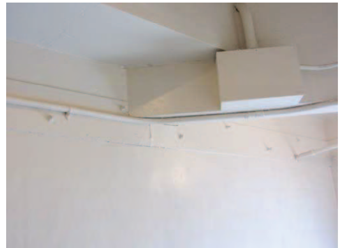
PICTURE 12 – Beam Framing and Anchorage Plates Along Wall
