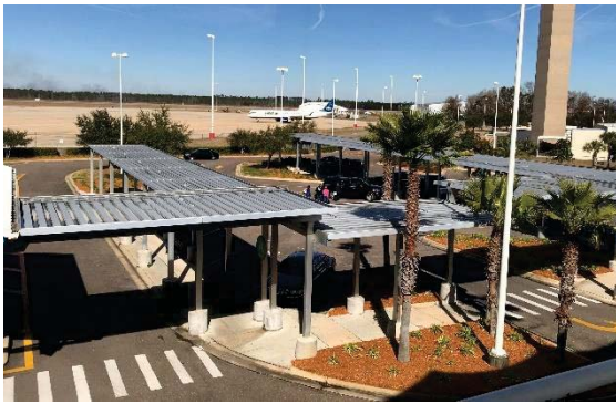
Premier Parking Lot
