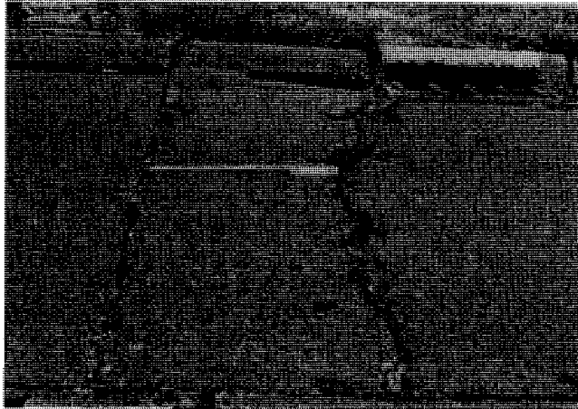
FIG. X2.35 Low-Severity Punchout
