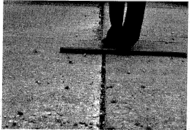
FIG. X2.13 Low-Severity Faulting
