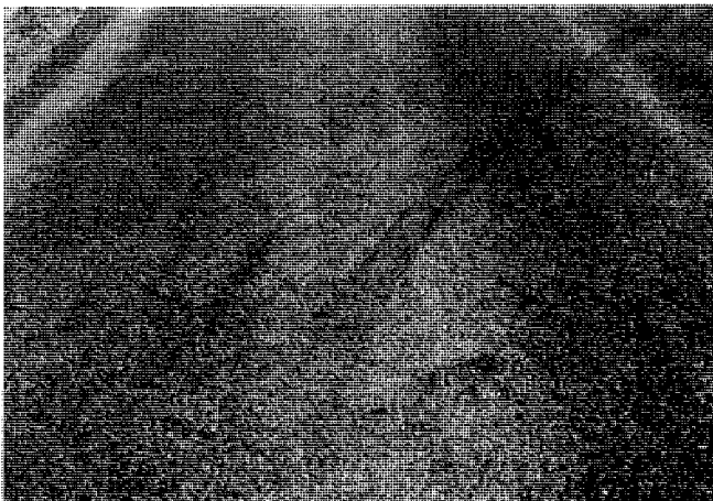
FIG. X1.4 Low-Severity Bleeding
