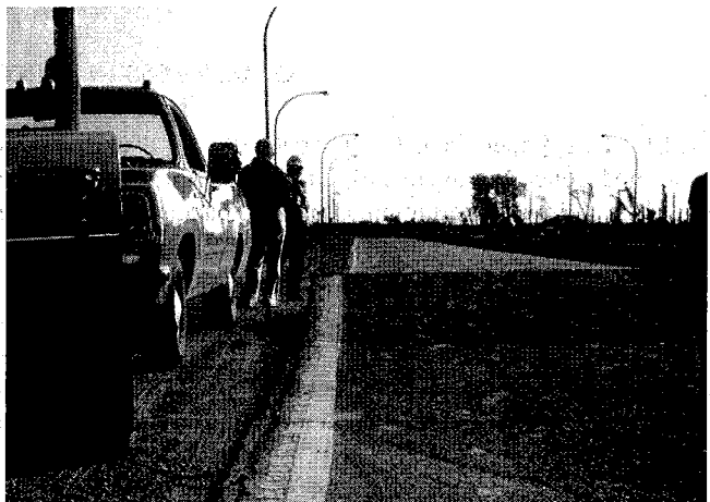
FIG. X2.3 High-Severity Blowup/Buckling
