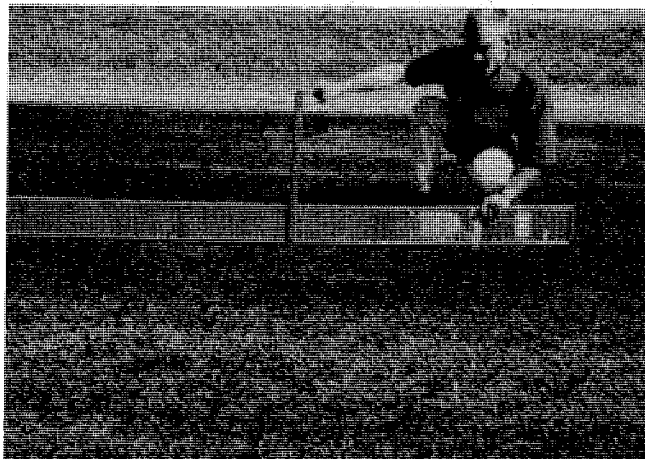
FIG. X1.16 Low-Severity Depression
