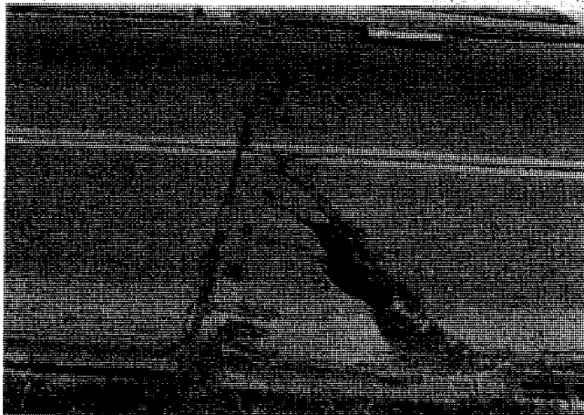
FIG. X2.36 Medium-Severity Punchout
