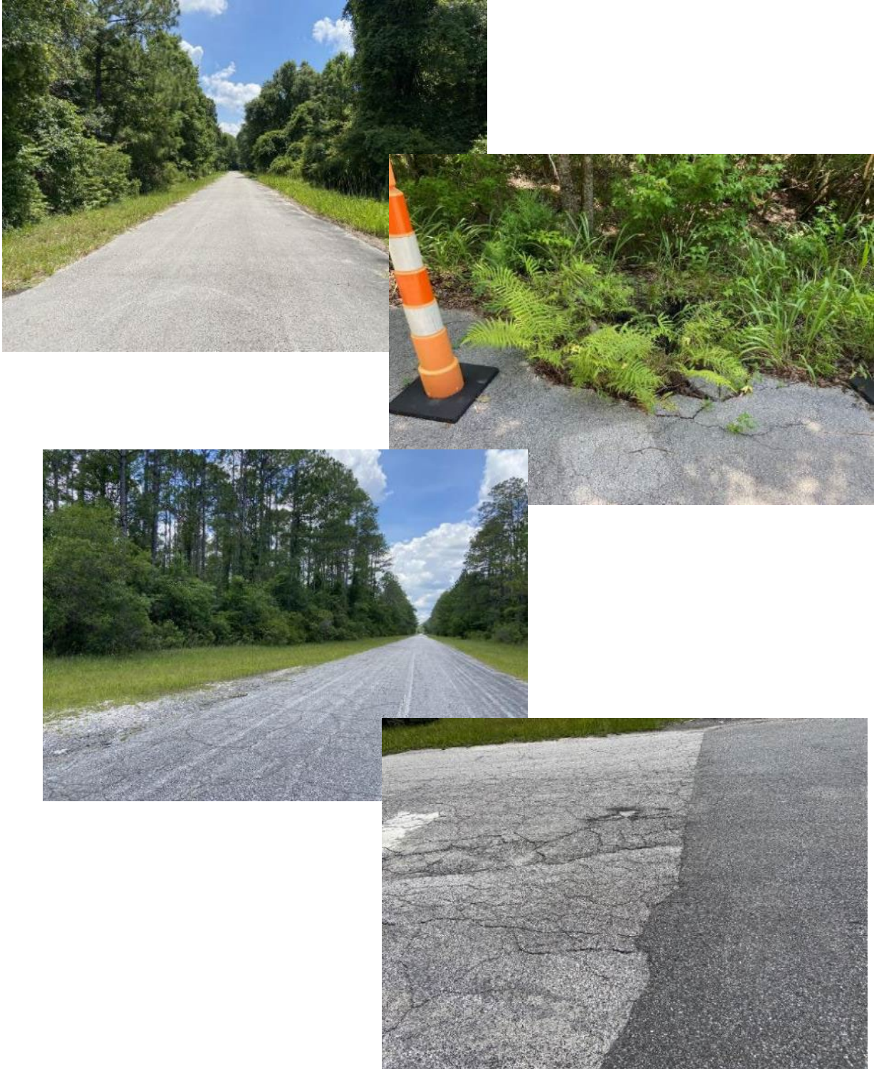
FIGURE 1-2: EXISTING EASTSIDE AIRPORT ACCESS ROAD CONDITIONS
