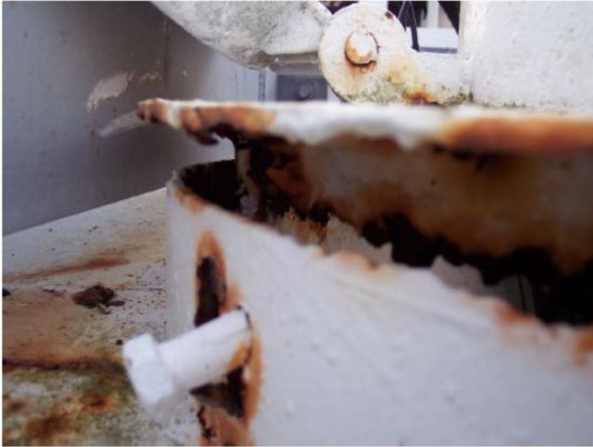
Corrosion at Top of Access Tube
