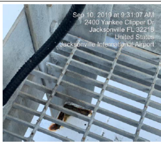
Figure 6: Typical Surface Rust at Post / Baseplate
