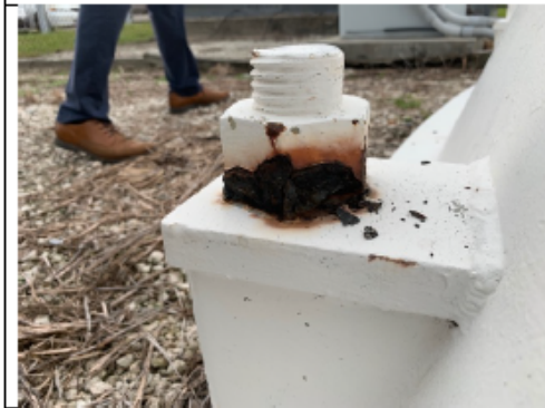
Figure 7: Typical Minor Damage to Bolts or Nuts That May Warrant Replacement
