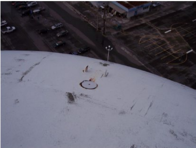
Roof with Corrosion at Cathodic Protection Cover Plate
