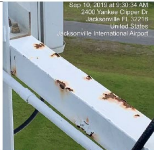
Figure 4: Typical Surface Rust on Catwalk
