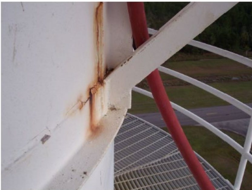
Antenna Balcony with Corrosion at Structural Member
