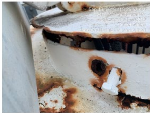
Figure 3: Damage to Roof Hatch – Recommend to Be Replaced
