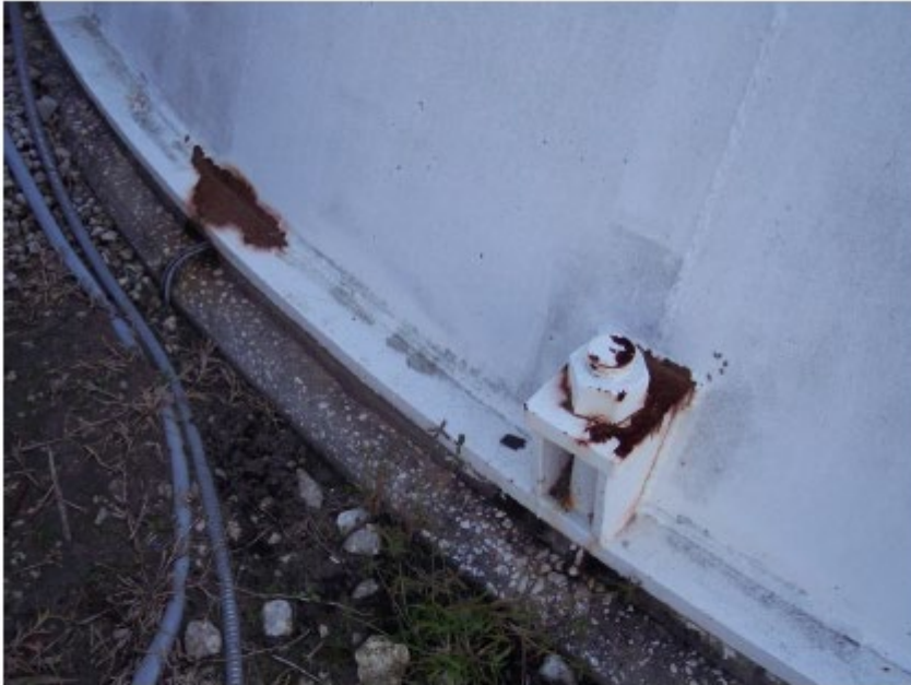
Corrosion at Tank Pedestal Foundation – base plate and anchor bolt
