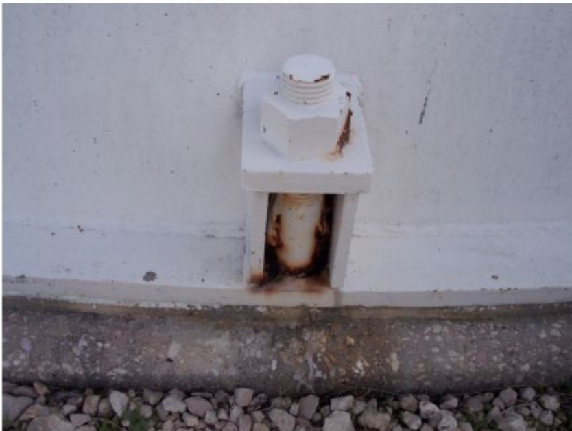
Anchor Bolt Corrosion
